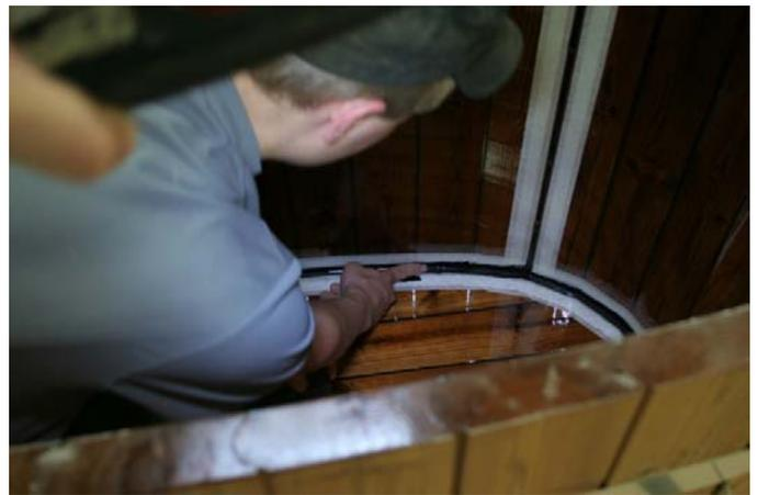
Smear out the sealant in the bottom seam with a finger. **TIP! You can use a disposable glove instead.**
