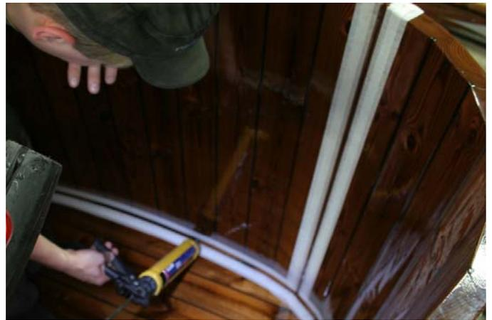
Apply sealant in the bottom seam.
