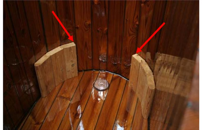
Place the first bit at the slat as the picture shows. Fasten all pieces in the sides.
