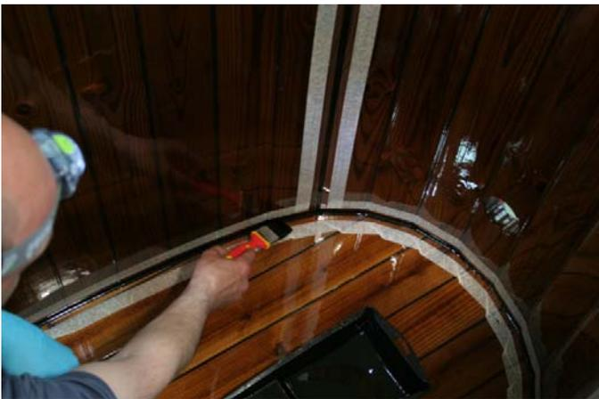
Apply TubCoat over the seams in the base and sides.
