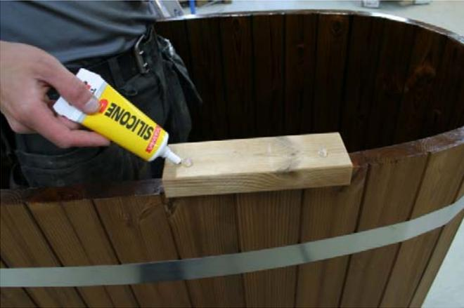
**Assembly of seat.** Use silicone in the holes before attaching them. That way you ensure water will not leak into the hole the screw makes.
