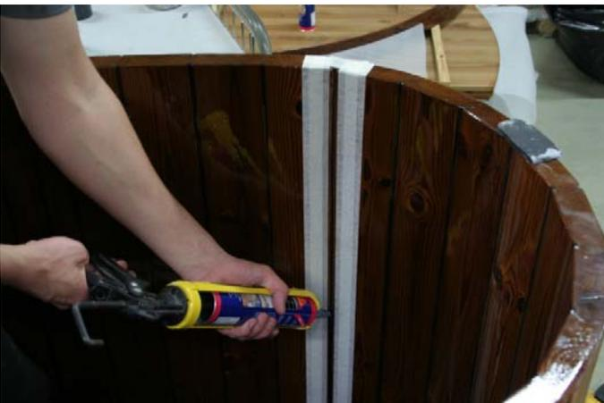
Apply sealant in the side module seams.
