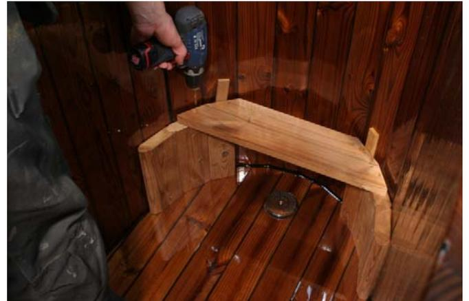
Pre-drill with 3mm drill and screw the seat in place with four screws. **Don't forget to use the included washers!**
